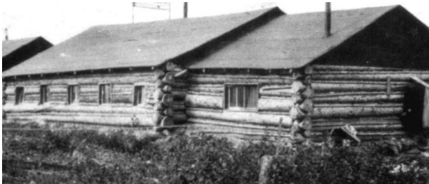
Trowsse Log House on George Street
